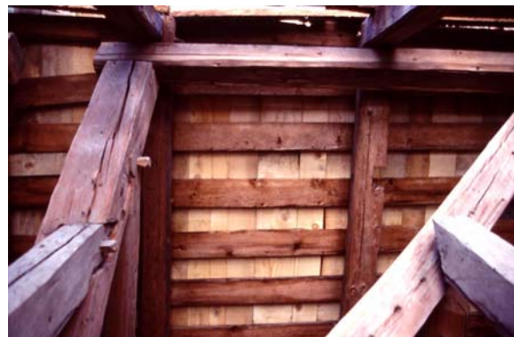
Fig. 4-5: Renovation example at Peiden Bad Church (Grisons, CH). Interior space after renovation: the old wooden shingles were replaced by roof boarding consisting of untreated boards. Photos: E. Mühlethaler, M. Lutz
