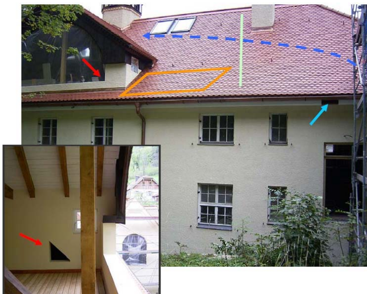
Fig. 4-7: Renovation of a power station and a residential building in Aschau (Bavaria, D.) The situation after the renovation in 2004 (rear side view of the building). Green: boundary between the residential area (left) and the bat area (right). Dashed blue line: former flight path for the ingress and egress opening. Light blue arrow: newly made opening that was not known to the animals in the previous year (2003) and which they do not use. Red arrows (large and small picture): additional opening on the roof terrace (there had been a large opening in the roof here in 2003). This which was accepted by the animals. Orange: unused space providing an access passage between the new opening on the balcony and the bat area, and skirting the residential area. Photos: A. Zahn
