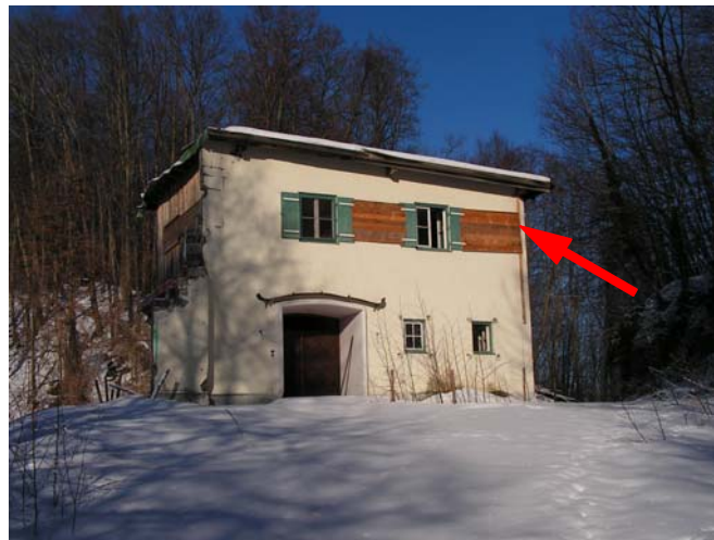
Fig. 4-12: Factory canteen, Murnauer Moos (Bavaria,D). Between the windows bat boards were fitted. So far they have been accepted only by a few individual animals. The colony still resides behind the soffit, as before. Photo: B. Wimmer
