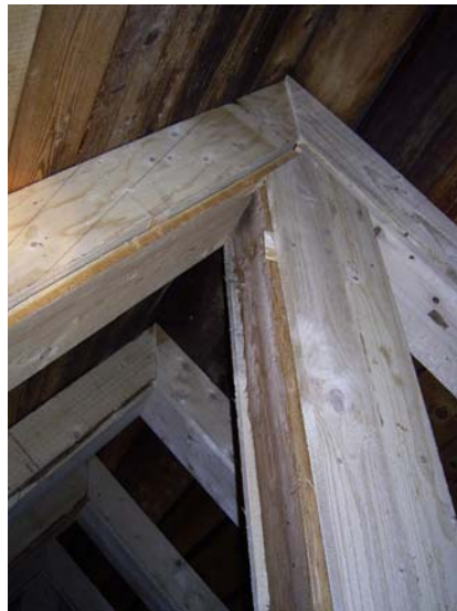
Fig. 4-27: In Au (Bavaria, D) load-bearing beams at the hanging places were covered with waste boards as a protection against droppings and urine. The animals were already hanging from the new boards in the first year, even though they preferred the hanging places located on the old roof laths. Photo: Andreas Zahn
