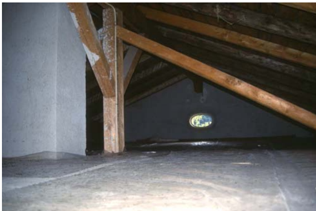
Fig. 4-8: Renovation example Primary School in Wald in Pinzgau (Salzburg, A). Thermal insulation was fitted on the roof space floor instead of the roof itself. The insulation boards were covered with a sheet to catch the droppings; in the background you can see the round egress opening. The external scaffolding was accepted by the animals. Photos: M. Jerabek
