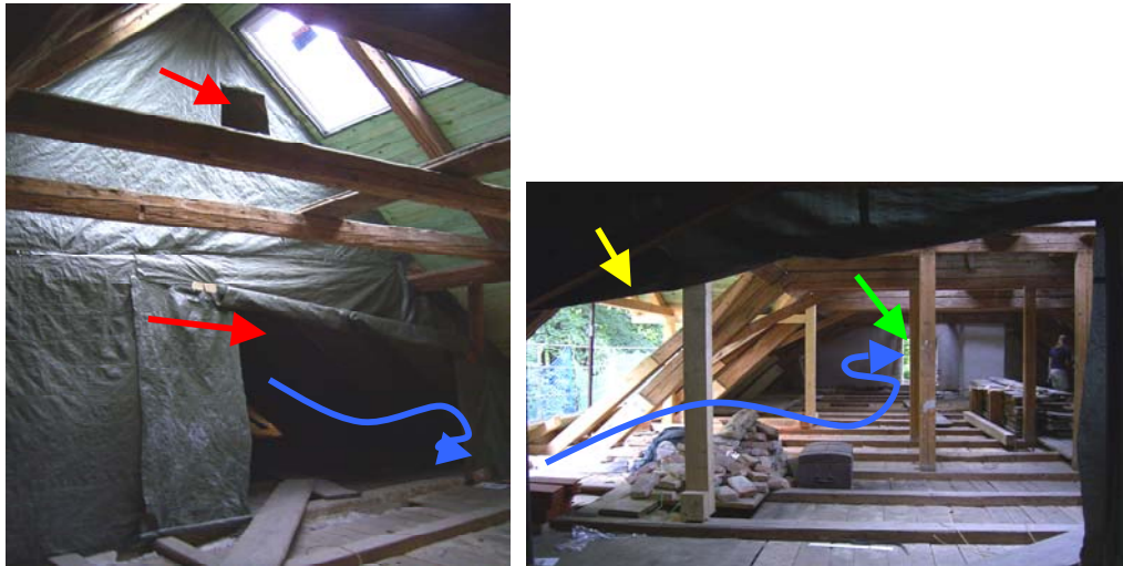
Fig. 4-6: Renovation of a power station and a residential building in Aschau (Bavaria, D.) The bat area is temporarily screened off using sheeting (picture on the left), with an open passage for incoming and outgoing access (red arrow on top) and an area open only during the night (red arrow at the bottom). The residential area to-be (picture on the right), seen from the bat area, with the future roof terrace opening (yellow arrow), and the original egress and ingress opening (green arrow). The animals' flight path towards the opening is marked by blue arrows. Photos: A. Zahn
