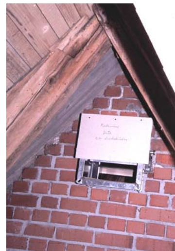
Fig. 4-26: In Beyharting (Bavaria, D) a vapour-permeable sheet was fitted along the ridge, making it possible for a certain amount of warm air to build up. Under the sheet there is boarding, from which the animals hang in summer, just as they did before renovation. If it is cold however (in spring), the animals roost in an adjacent roof frame with higher temperatures, which is also as it was in previous years. For this purpose they fly through a fire retarding flap (small picture), which was fitted about 70 cm below the former transit passage (a hole in the wall). Photos: A. Zahn
